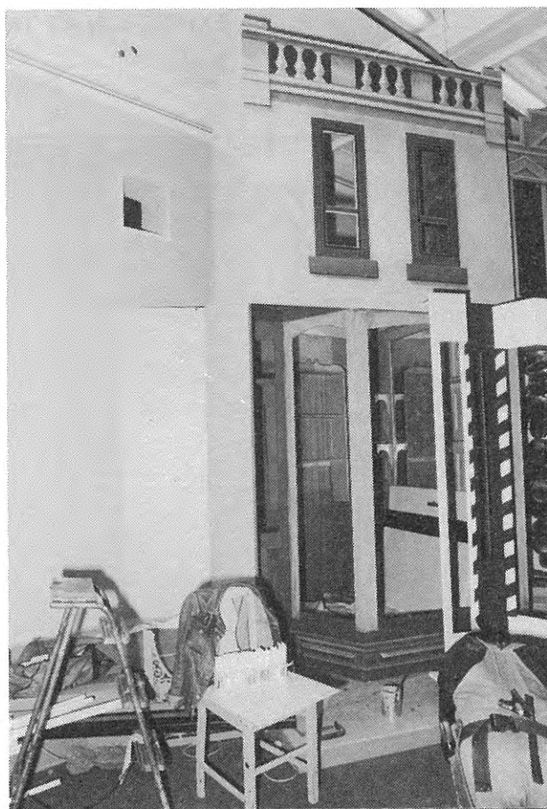
On Saturday, two days before the opening, construction work was still underway. Painting, carpentry, the installation of sound and lighting, the placement of objects and the positioning of perspex all came together finally, and by the time the first guests arrived no-one would have guessed the previous rush.
