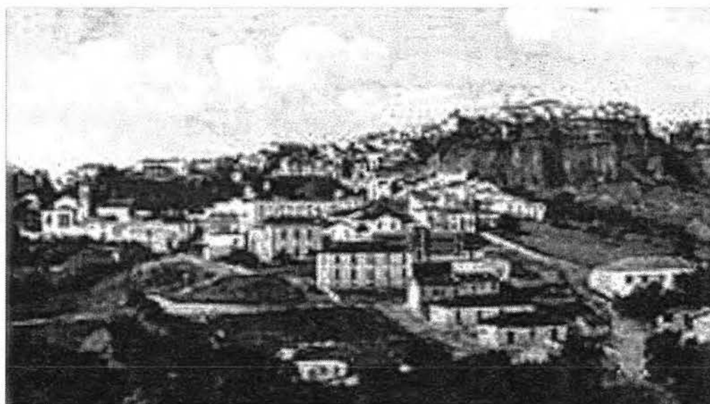
View of the Town of Caulonia, c. 1960.
